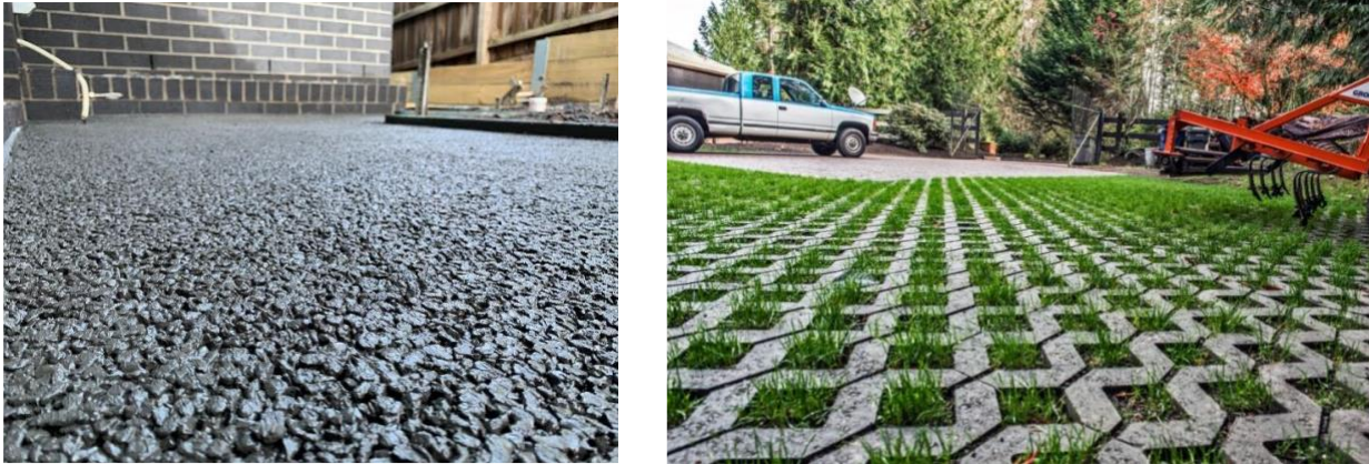
Figure 32: Porous Concrete (left) and a Plastic Grid System (right) (Permeable Concrete 2022)
