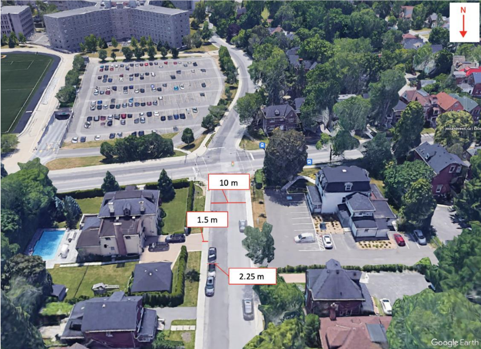
Figure 44: Current Cross-section Dimensions for Albert St. (Sidewalks are the same dimension on both sides) (Google Earth 2022c)
