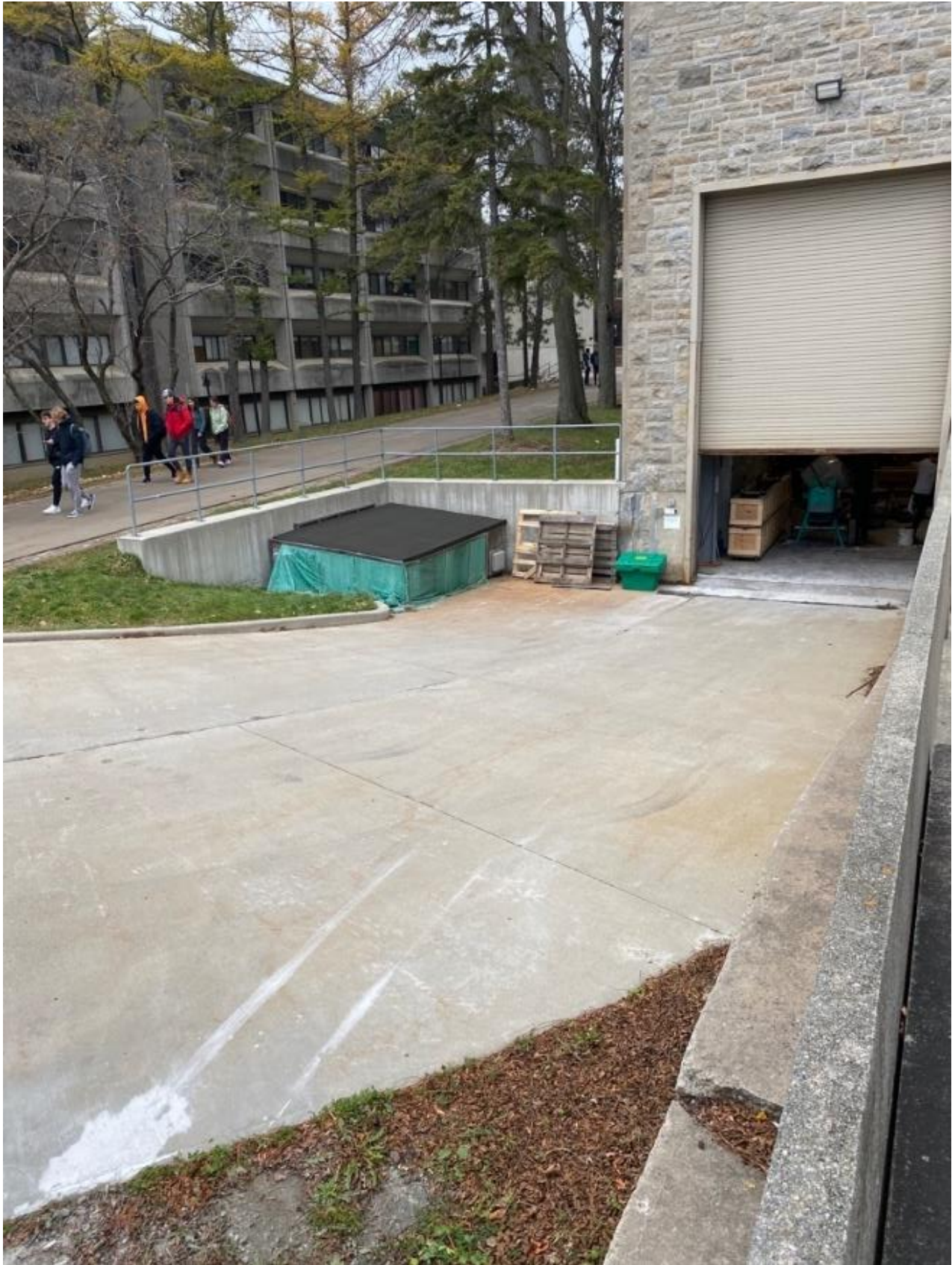
Figure 42: Photo of the Ellis Hall Dock Door ramp at Site #2
