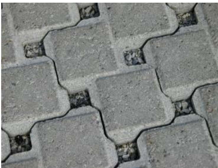
Figure 19: An example of the permeable pathing design used to improve infiltration (Sustainable Technologies 2019)
