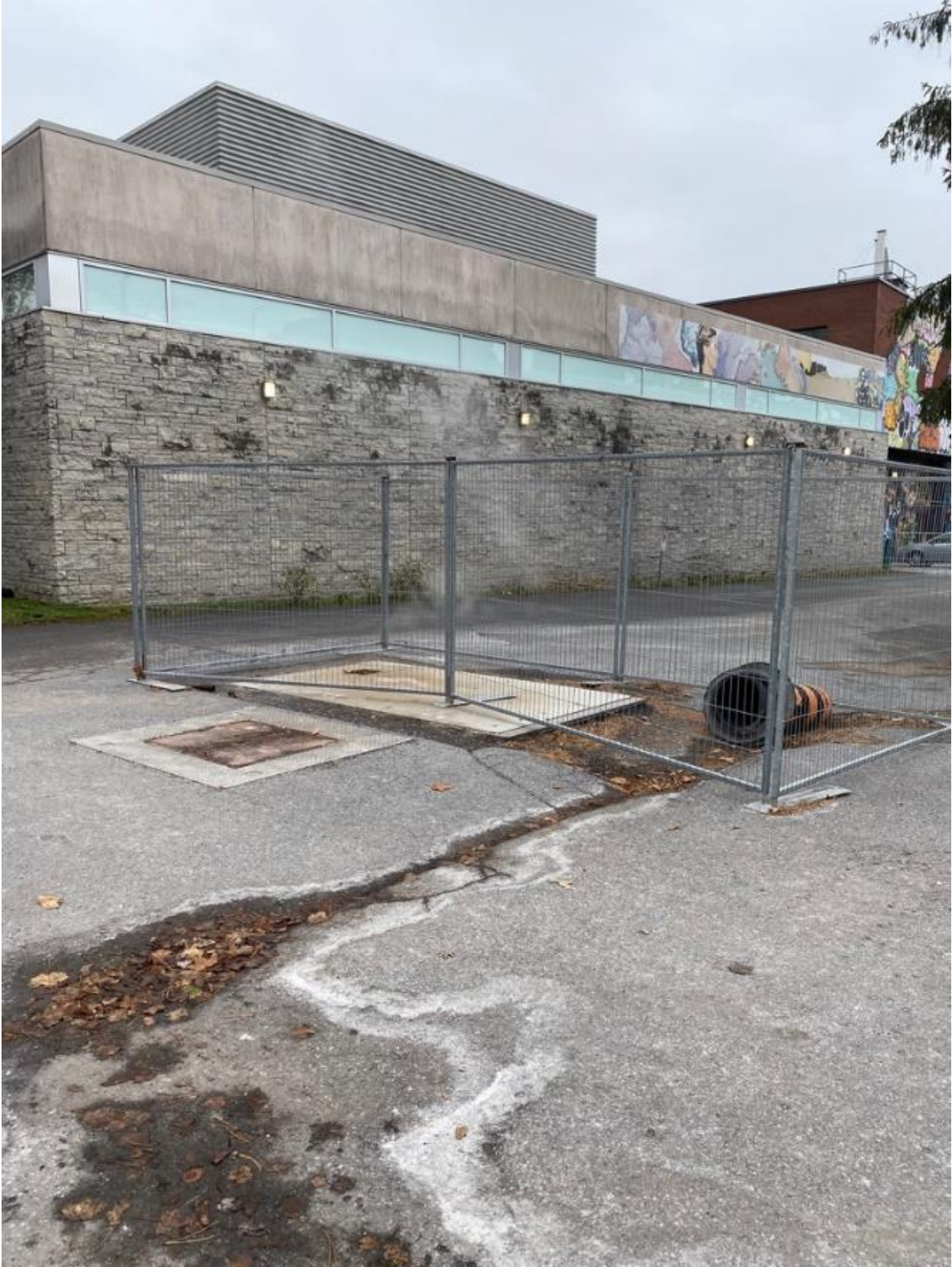
Figure 39: Photo of the fenced off grates in the middle of Site #2.
