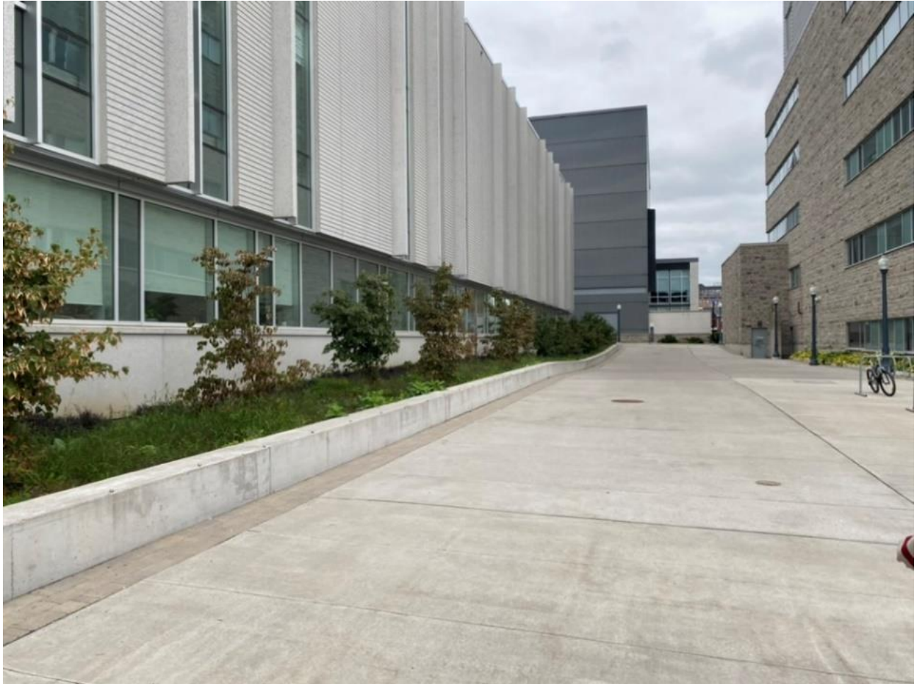
Figure 51: Photo of the East walkway beside Mitchell Hall (Site #4).
