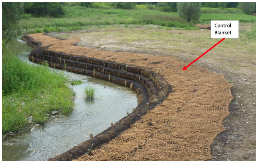
Figure 11: Example of a Natural Fiber Erosion Control Blanket in use (Devtron Sale Ltd 2022).
