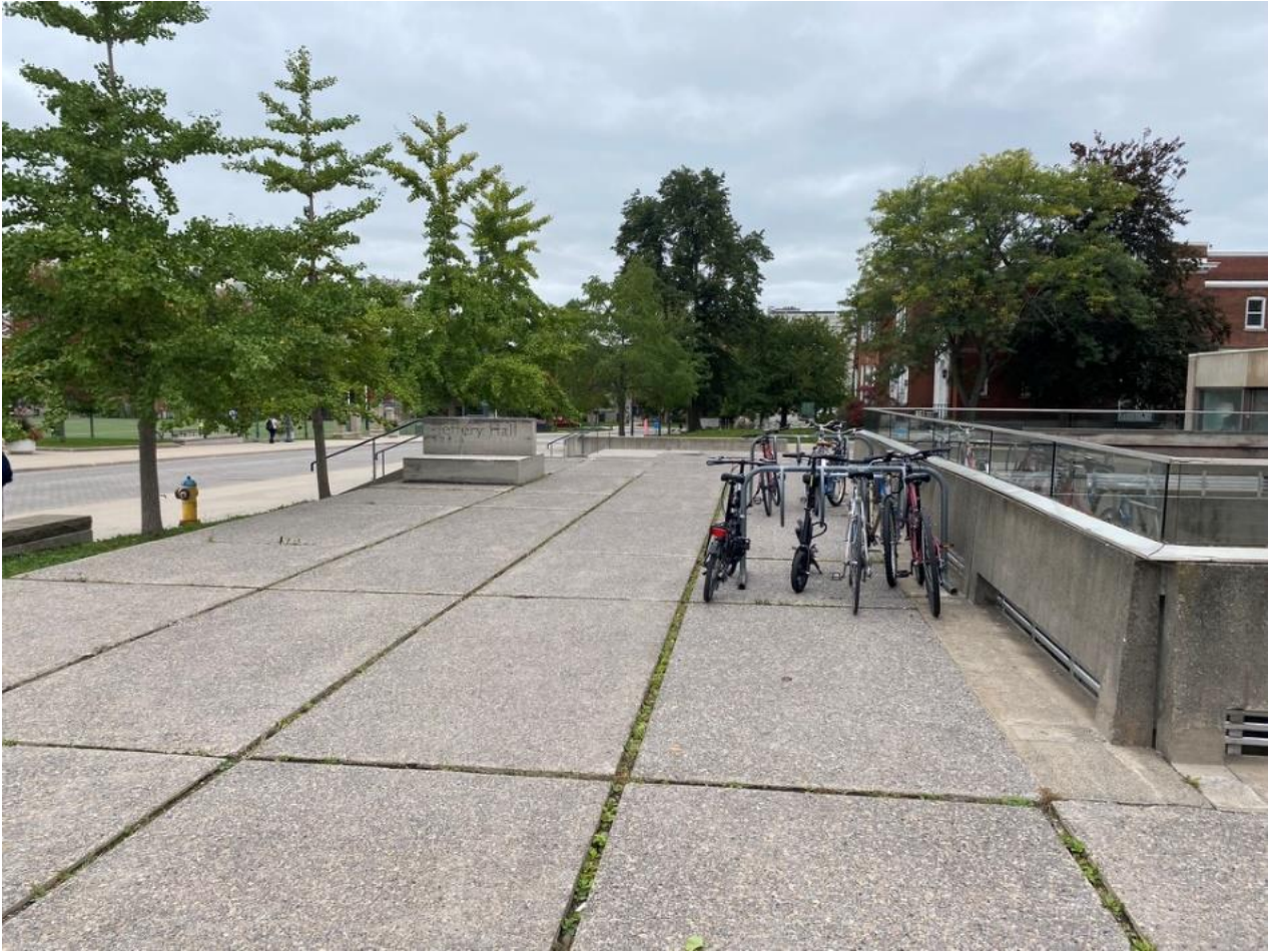
Figure 46: Photo of the East entrance area of Jeffery Hall (Site #3).
