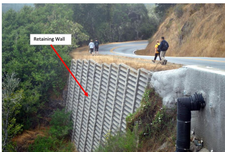
Figure 15: Example of a crib retaining wall (Norwegian Geotechnical Institute 2016).
