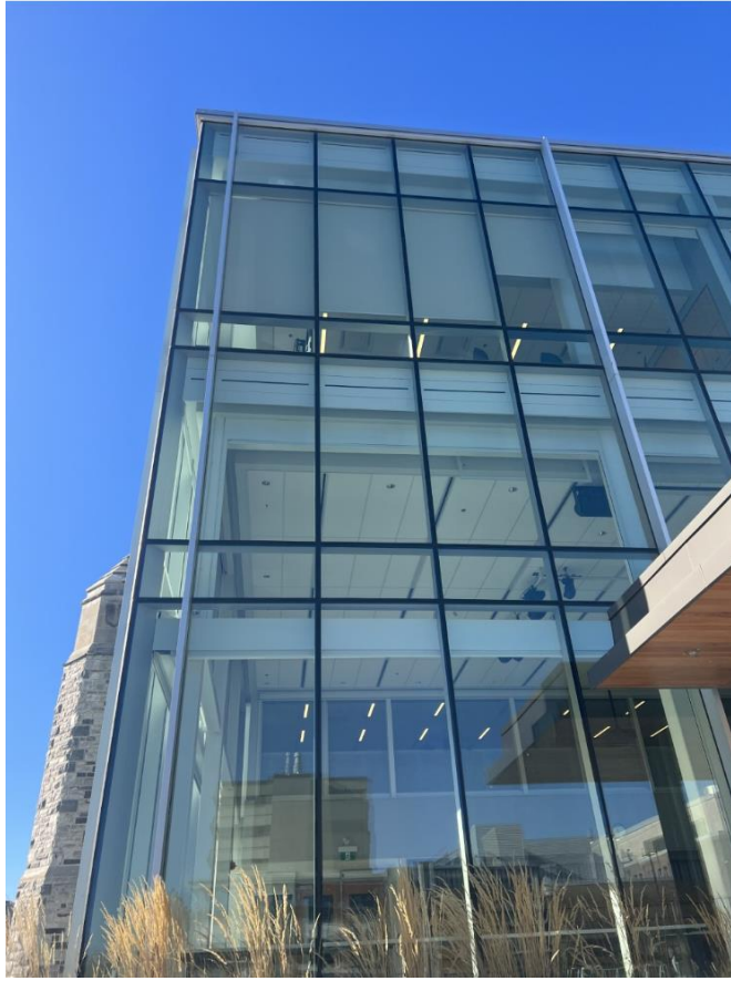
Figure 4: Mitchell Hall's glass curtain walls as seen from outside.
