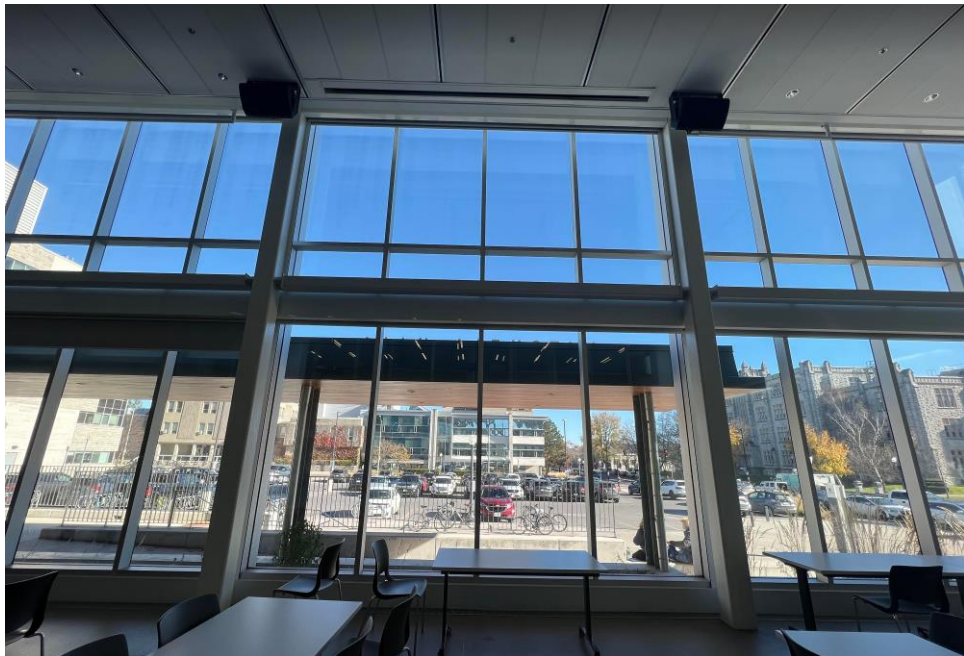
Figure 5: Mitchell Hall's glass curtain walls as seen from inside.
