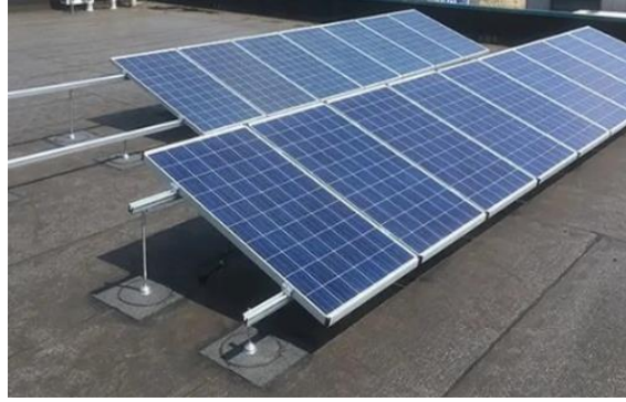
Figure 11 Attachment installation (Solar System 2022)
