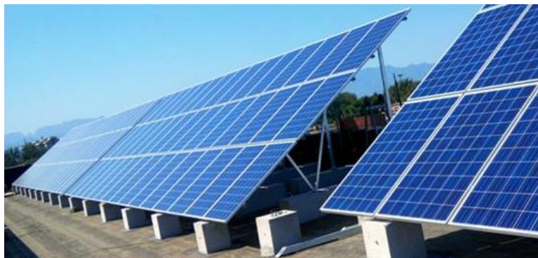
Figure 12 Foundation system (Solar First n.d.)
