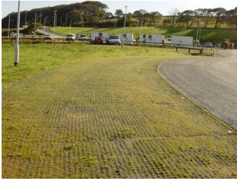
Figure 7-2 Examples of possible driveable greening infrastructure that utilizes structural load bearing components below grade, allowing vegetation to grow unobstructed at the surface.
