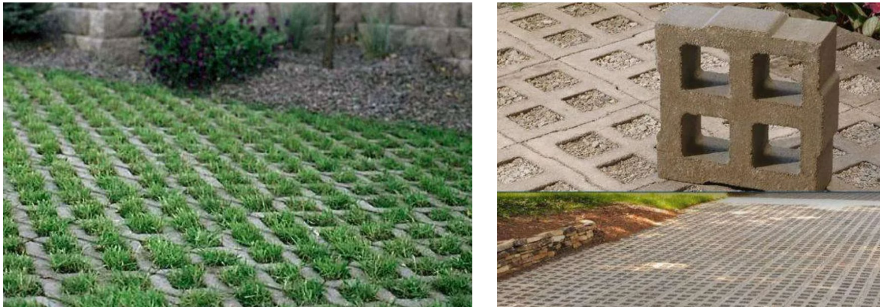
Figure 7-1 Examples of possible driveable greening infrastructure that integrates vegetation and concrete pavers at grade.
