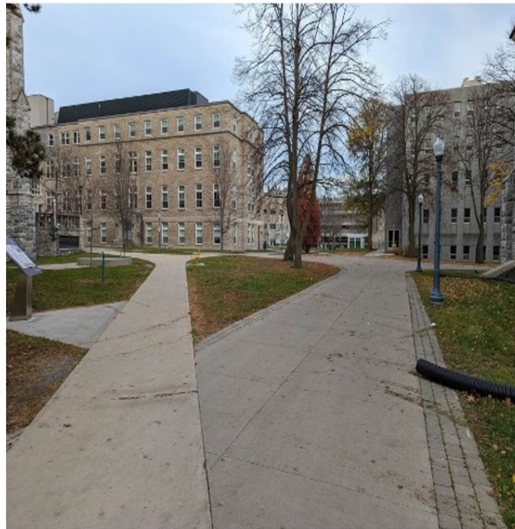
Figure 6-7 Existing condition of pathway network south of Douglas Library.
