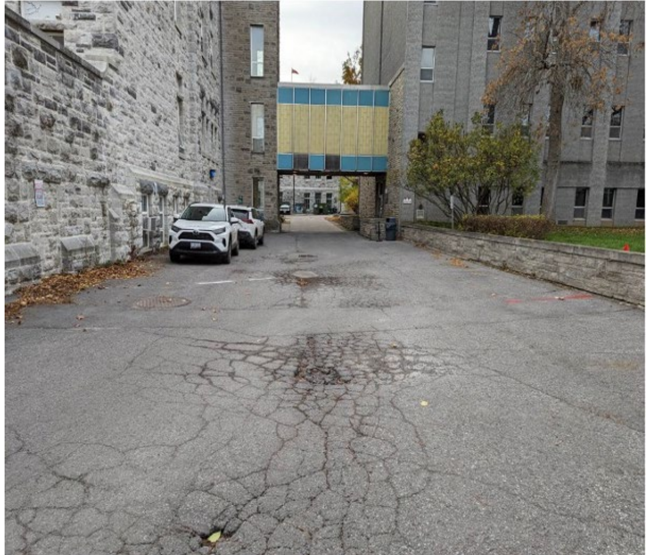
Figure 6-3 Existing condition of area between Clark Hall and Fleming Hall.
