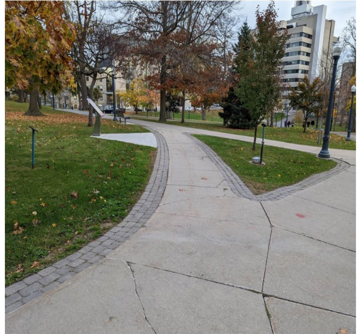
Figure 6-11 Existing condition of pathway cut-through east of Theological Hall.
