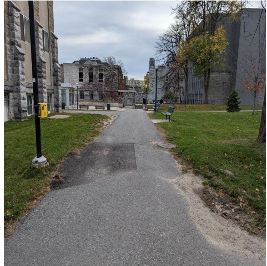
Figure 6-8 Existing condition of pathway west of Nicol Hall.
