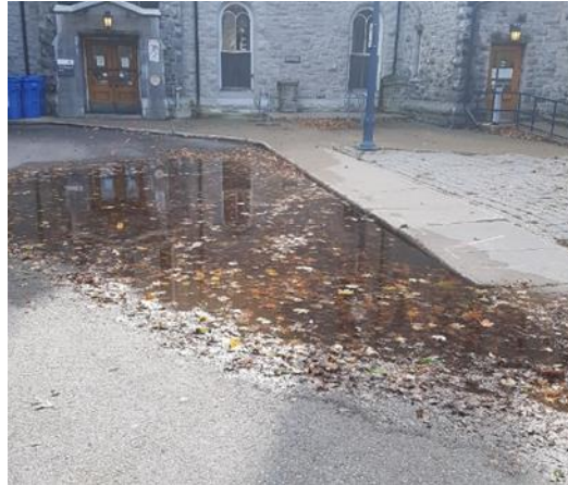
Figure 12: Pooling at the Back Entrance of Theological Hall (credit for photo: Matt Grekul)
