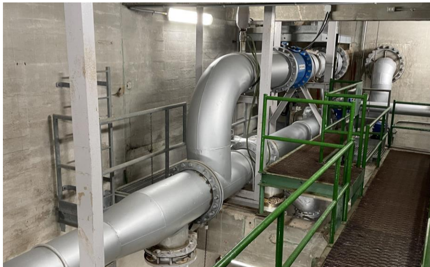
FIGURE 2: DISPLAYS WHERE THE TEAM PLANS TO INSTALL THE HEAT EXCHANGERS IN THE PUMPHOUSE.
