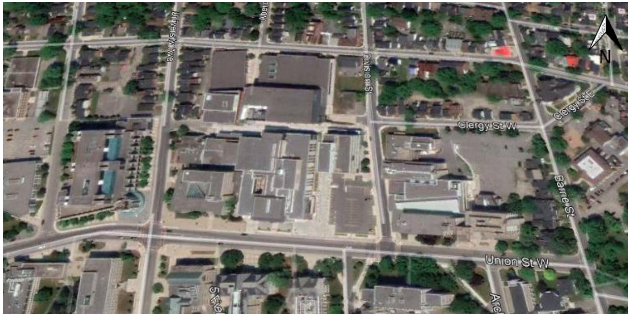
Figure 20: Current site conditions of North of Union Precinct Area (Google Earth, 2019).
