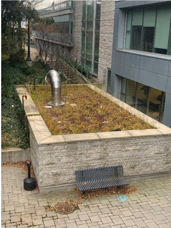
Figure 8: Botterell Hall green roof; image taken by Greengenuity (11/13/2020).
