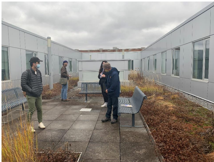
Figure 12: Goodes Hall intensive green roof; image taken by Greengenuity (11/13/2020).
