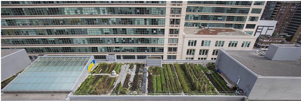
Figure 21: Ryerson University urban farm green roof (Ryerson Urban Farm n.d.).
