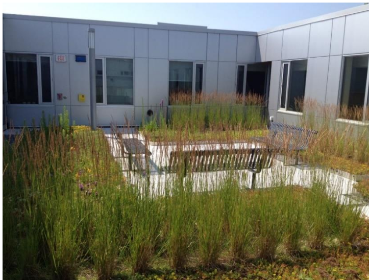
Figure 1: Existing green roof on Goodes Hall (Queen's University Sustainability Office, n.d.).
