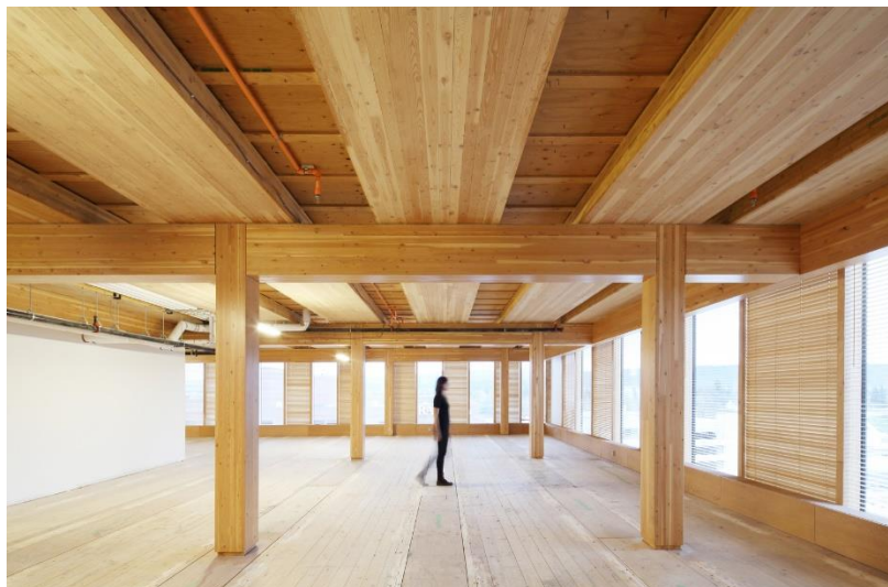
FIGURE 11: COLUMN AND BEAM SYSTEM (“GLULAM HANDBOOK VOLUME 1” 2013)
