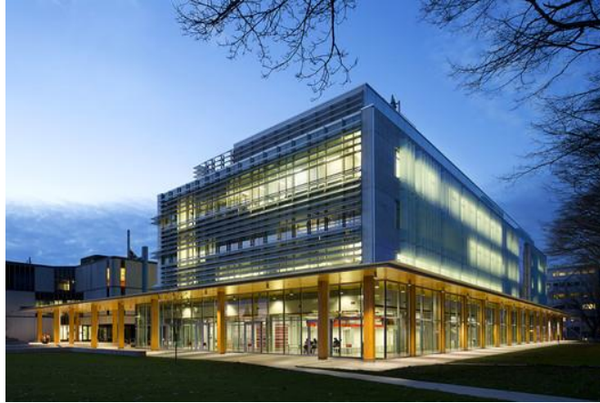
FIGURE 5: UNIVERSITY OF BRITISH COLUMBIA EARTH SCIENCES BUILDING (ARCH DAILY 2023)
