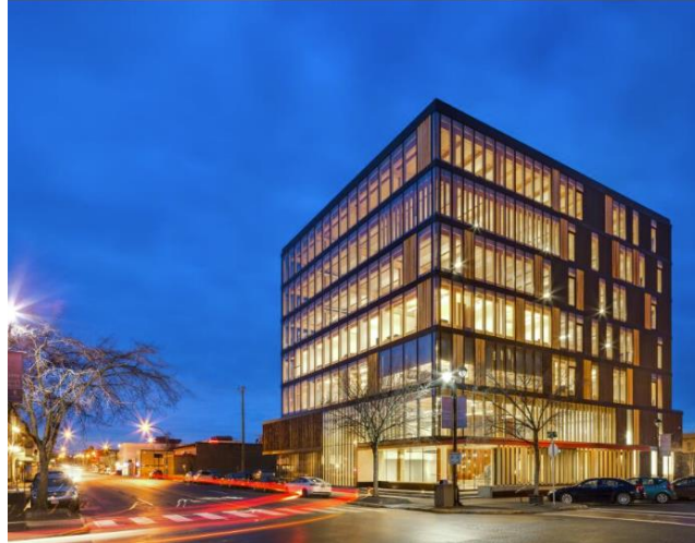
FIGURE 4: WIDC BUILDING IN BRITISH COLUMBIA (WOOD-WORKS N.D.)
