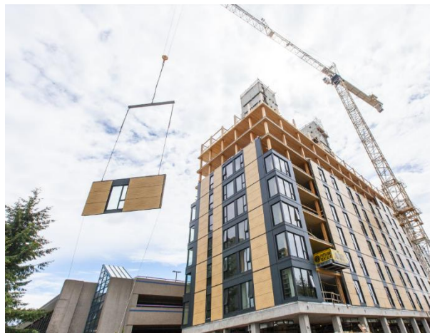
FIGURE 2: CONSTRUCTION OF THE BROCK COMMONS BUILDING (WOOD-WORKS 2017)
