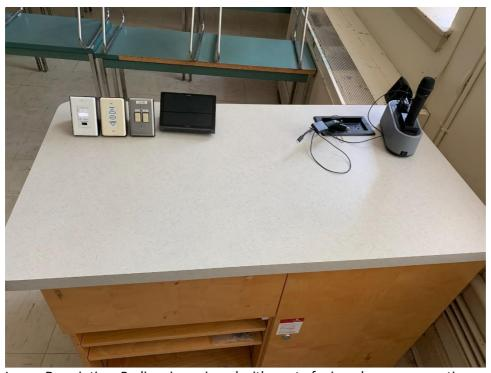
Image Description: Podium is equipped with a set of microphones, connection cords to present media, lecture capture as well as lighting control for the room.
