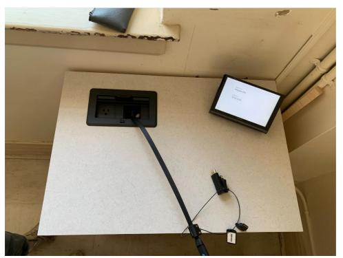
Image Description: Small podium is equipped with a set of connection cords to present media as well as volume control.
