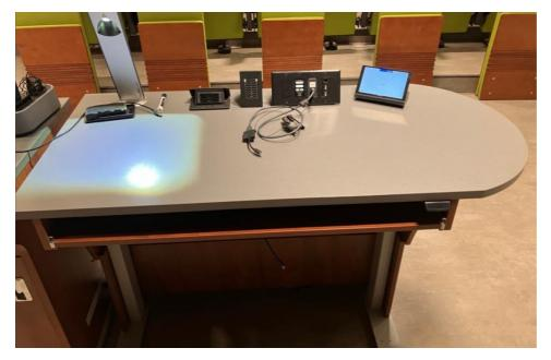
Image Description: Top down view of the podium. This podium is equipped with a set of microphones, a document camera, lecture capture and wireless presentation. The podium is height adjustable.
