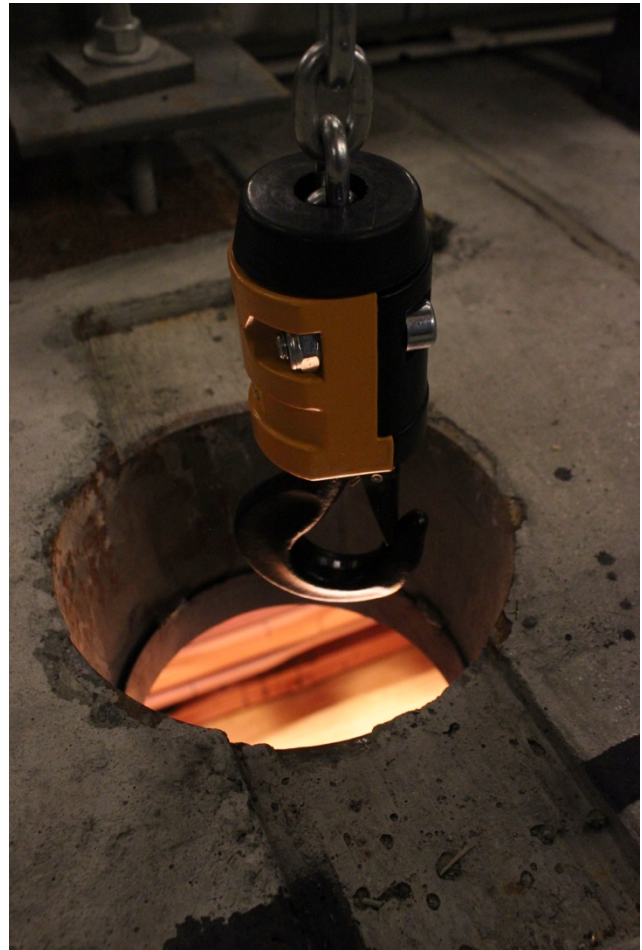
Figure 6 – Performance Hall Ceiling Rigging Hole (Kevin Tanner)
